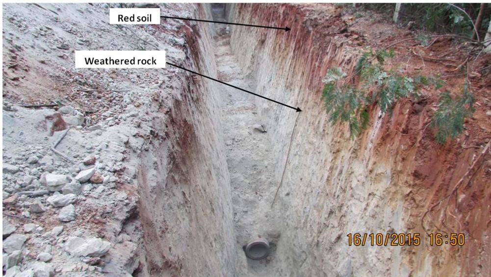
Figure 2. Trench excavated for the proposed pipeline project at the IISc Campus.
